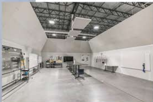
Modular freestanding partition walls fitted with acoustical hanging baffles to control noise transmission in an in-plant conference room
